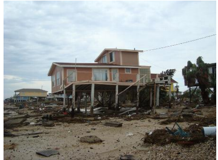
Lack of Dune Protection
